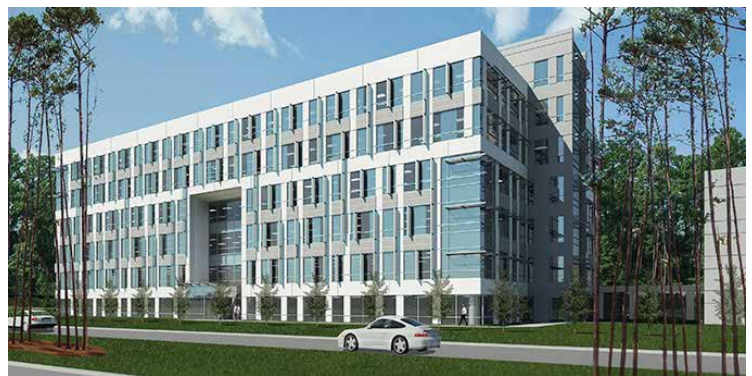
The savings realized during tilt-up construction provided the budget required for incorporating high end finishes in the lobby and other building areas. (Rendering courtesy of Powers Brown Architecture)
