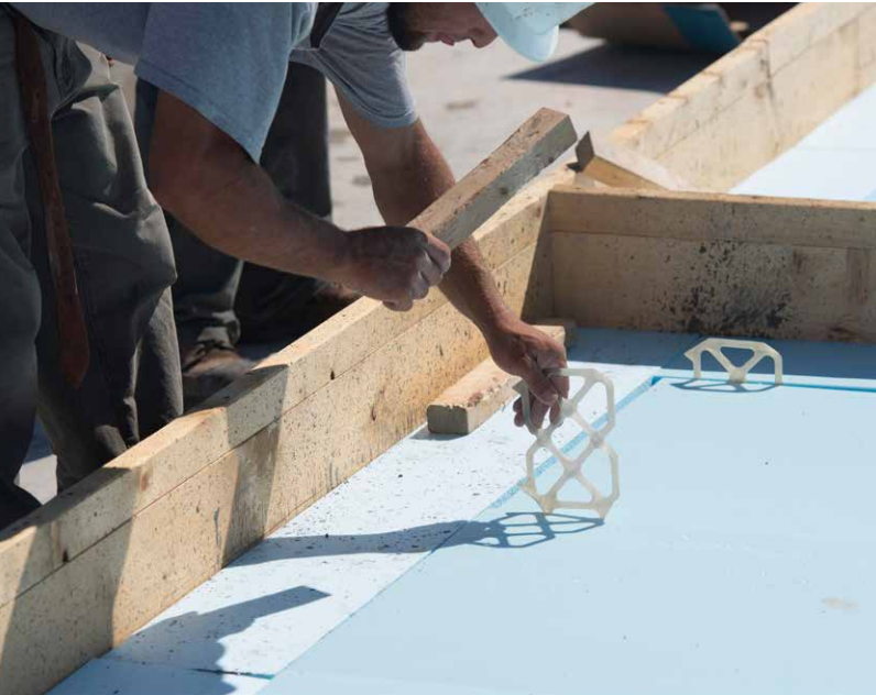
The Delta Tie is a two-dimensional truss of structurally non-conductive, non-corrosive, low thermal conductivity fiber composite used as a wythe connector for concrete sandwich panel construction. It installs quickly between insulation sheets.
