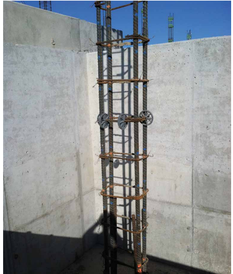
Plastic Spacer Wheels provide a simple way to center the rebar cage inside the concrete forms.
