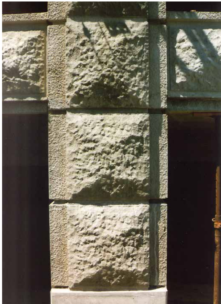
The cast-in-place concrete has deeply textured surfaces to deaden noise from a nearby concert stage.
