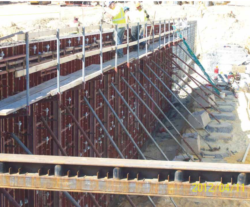
The Sym-Ply forming system includes a complete line of accessories, such as walkway brackets and braces.
