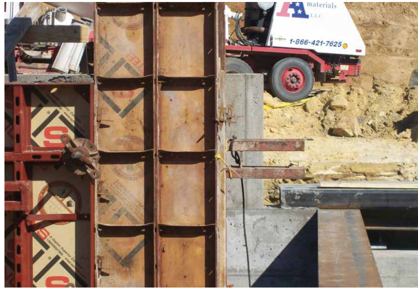
Standard Taper Ties can still be used even when Steel-Ply is included in a project, simplifying inventory.
