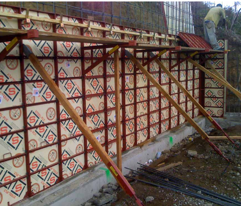
The forms and accessories are simple and easy to set up, providing a predictable load capacity and a safe work environment.
