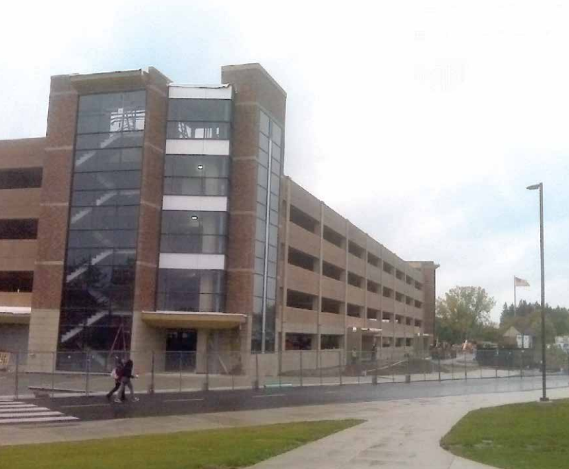
Compared to other construction methods, precast structures have a rapid schedule, and Sleeve-Lock helped maintain it.
