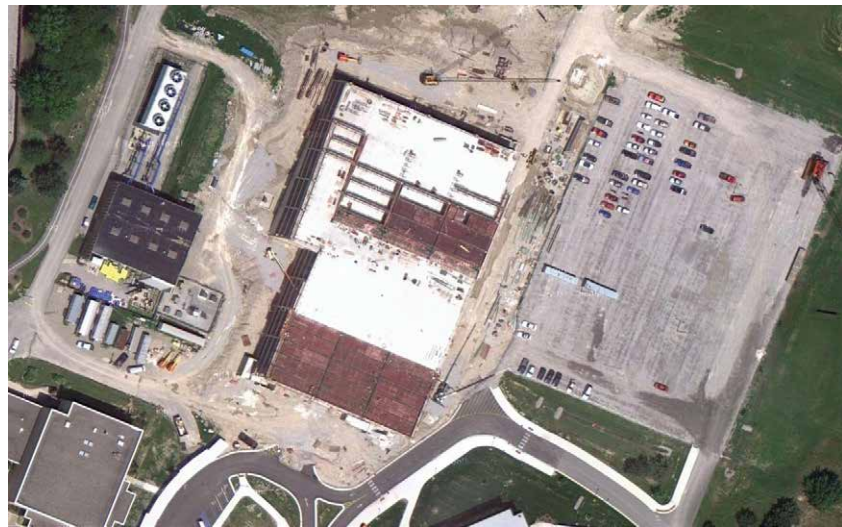
Satellite view of construction courtesy of Google Maps.
