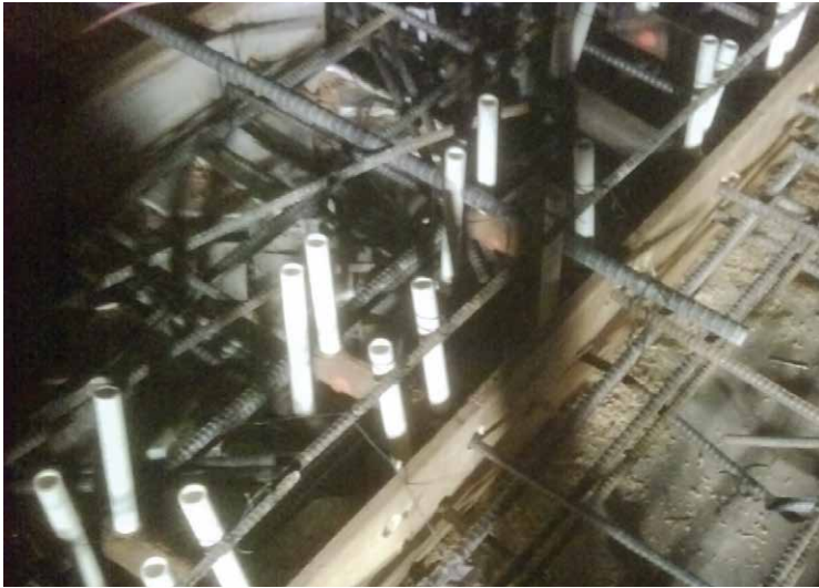
Sleeve-Lock is a full ultimate strength coupler that meets or exceeds building codes and self-centers for fast installation.
