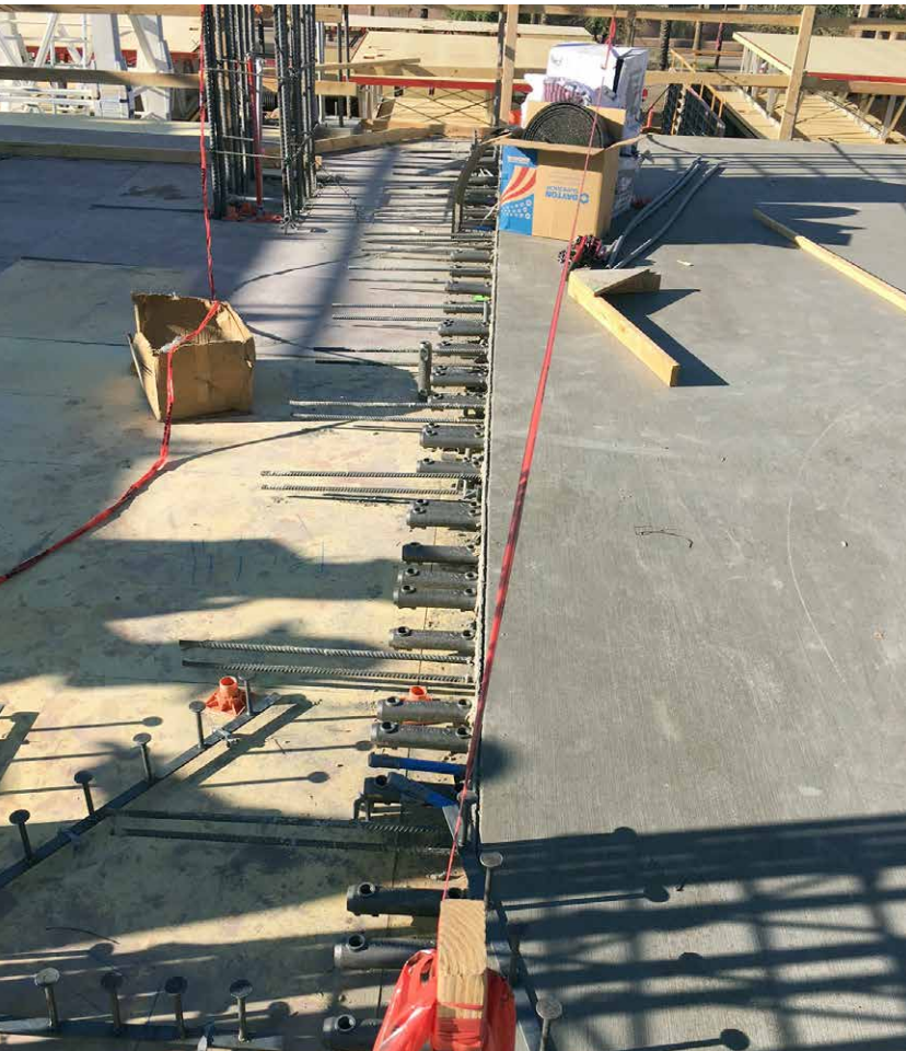
Sleeve-Lock grout sleeves were epoxied in place along the edge of a post-tensioned raised slab.
