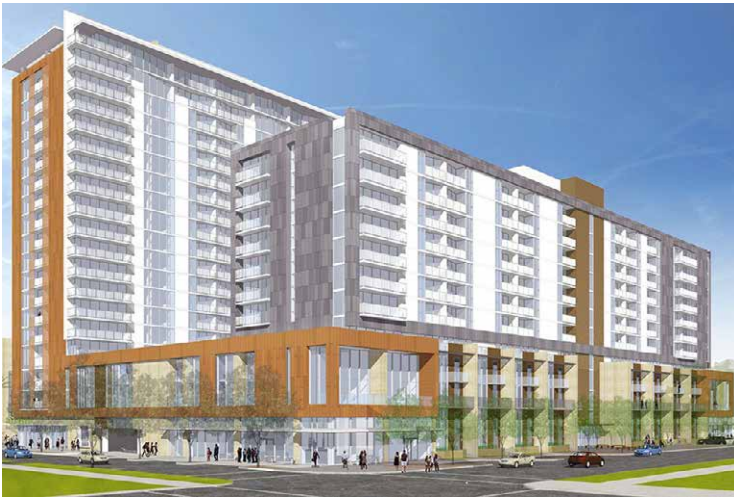
Delays due to unusually wet weather, NCAA games and holiday events in the area made finding ways to optimize construction time essential.
