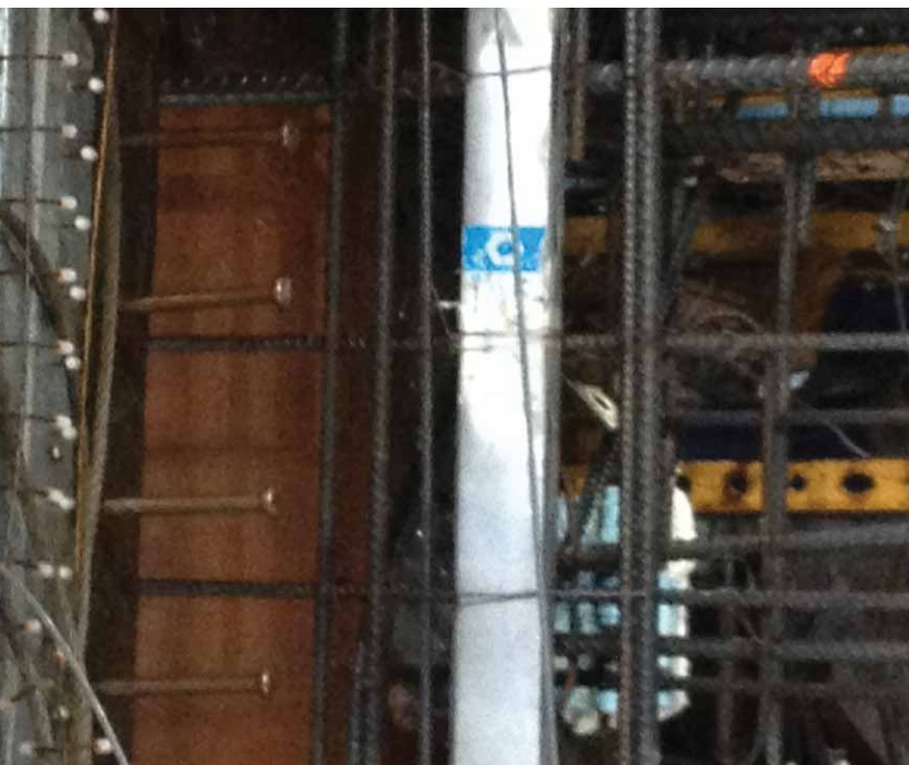
The concrete contractor chose D55 MetalStrip because they needed an engineered product solution for the core wall-to-slab connection that had a minimal on-site storage footprint, provided an easy installation to avoid construction delays and guarantee high-strength results.
