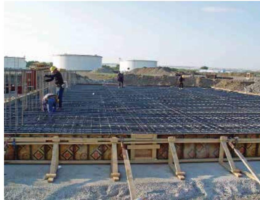
A new rail facility, electrical substation and control room featured concrete.
