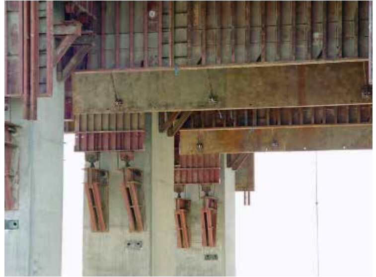
Column-mounted Anchor Brackets and self-spanning Max-A-Form capability eliminated conventional shoring.
