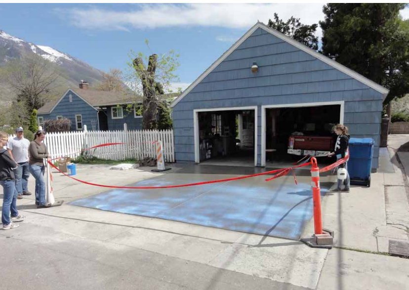
The students gained valuable hands-on experience with all steps in the process, including applying Cure & Seal 1315 J22WB.
