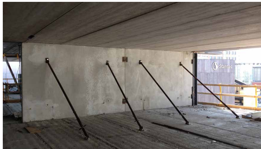
The load-bearing precast walls were aligned with braces.
