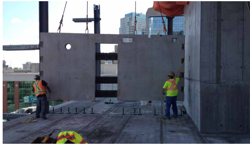
Walls were lowered onto Dowel-Ins tied to the previous level.
