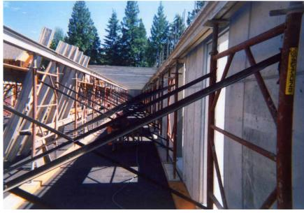
The contractor asked Symons for advice on shoring layouts and equipment for forming the slab above the parking garage.
