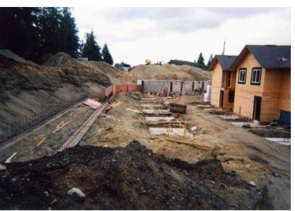
Interested in controlling concrete construction costs by eliminating job-built forms, the contractor decided to use Steel-Ply forms on this structure.
