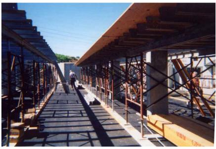
The strength of this heavy duty shoring system permits wide support spacings which allows the construction crew to move around freely.
