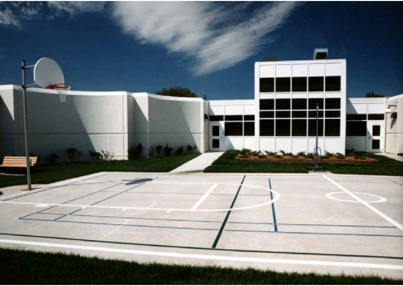
The wall surrounding this exercise area and gardens was created with a combination of Flex-Form and Steel-Ply components.
