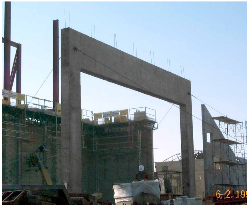
The contractor was impressed with the smooth finish of the proscenium arch.
