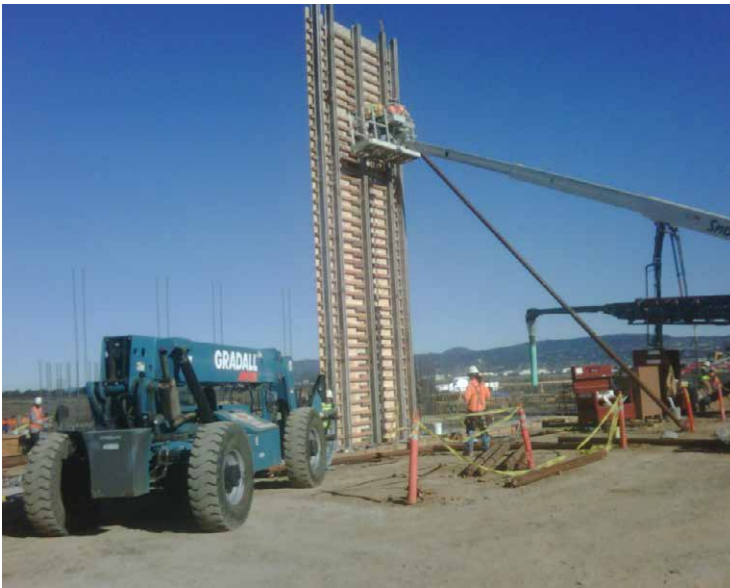
The initial crane lift of the form being set.
