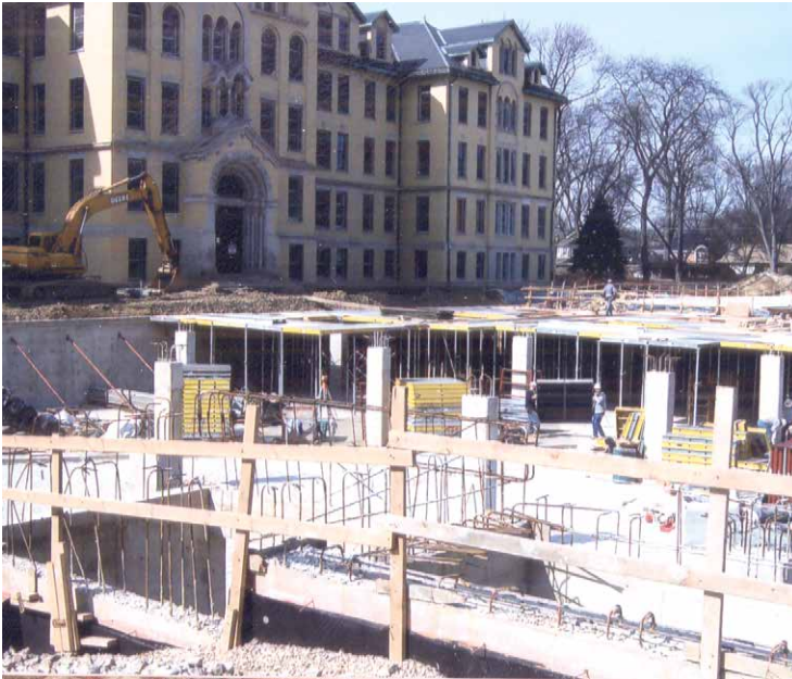
The drainage slope required in this project was easily accommodated by the DeckFast deck support system.
