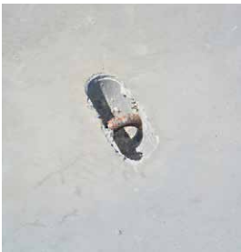
High capacity lifting anchors embedded in the panels provided strong lifting points.
