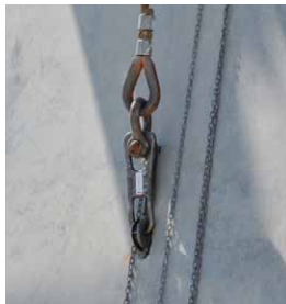
High capacity lifting anchors embedded in the panels provided strong lifting points.
