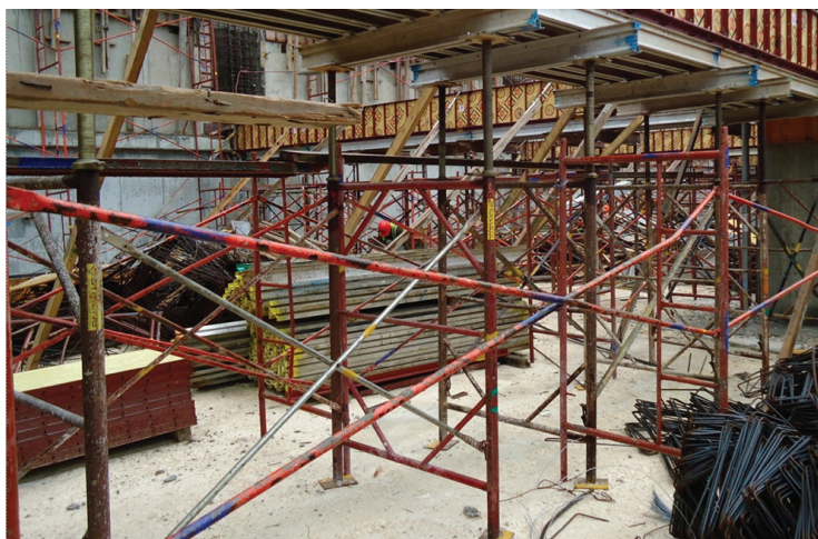
The FrameFast shoring system provided support for the concrete beam forms.
