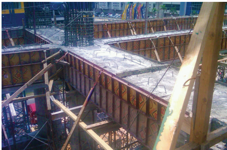
Steel-Ply was used in a horizontal configuration to form support beams for each floor of the mall and parking garage.
