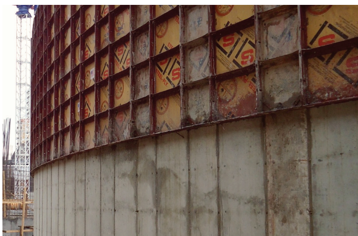
A combination of filler sizes allowed Steel-Ply to be set to a radius.
