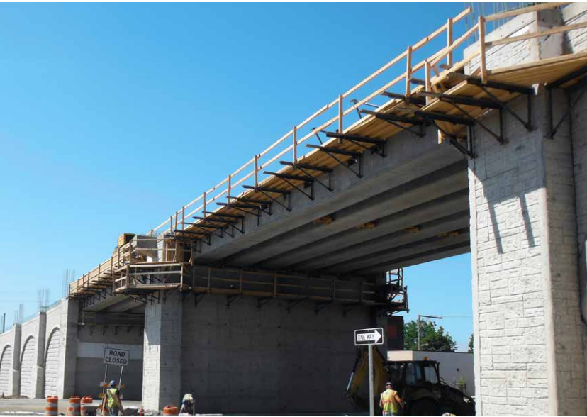
Using the Dayton Superior Century Series Bridge Deck Hanger helped avoid costly construction delays.
