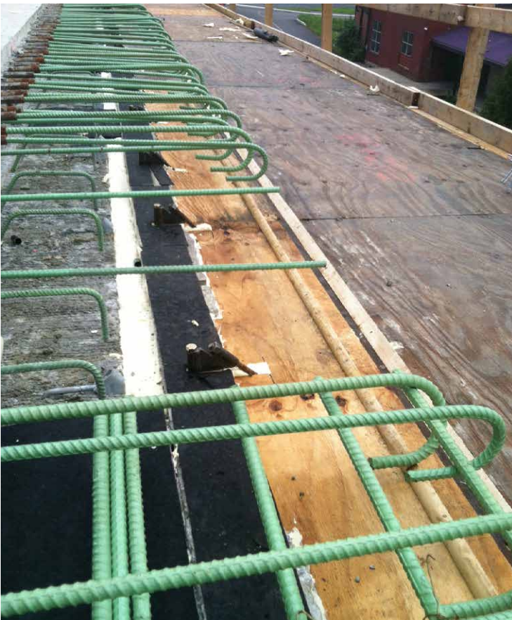
The Dayton Superior Century Series Bridge Deck Hanger installed in the 10th Street Bridge precast facade panel.
