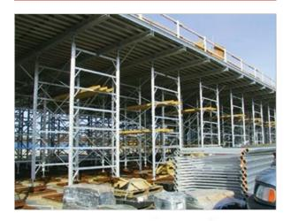
Hi-Lite 12K Shoring Frames are easily adjusted and attach safely and seamlessly to beams and stringers.
