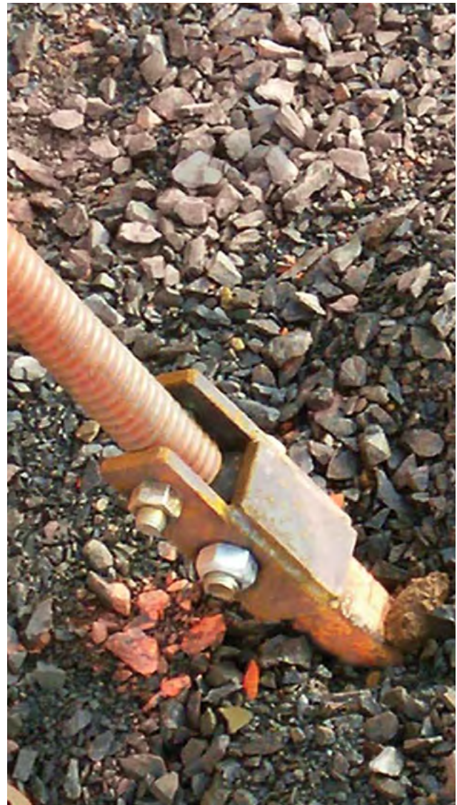
INCORRECT Brace-to-HGA Connection
