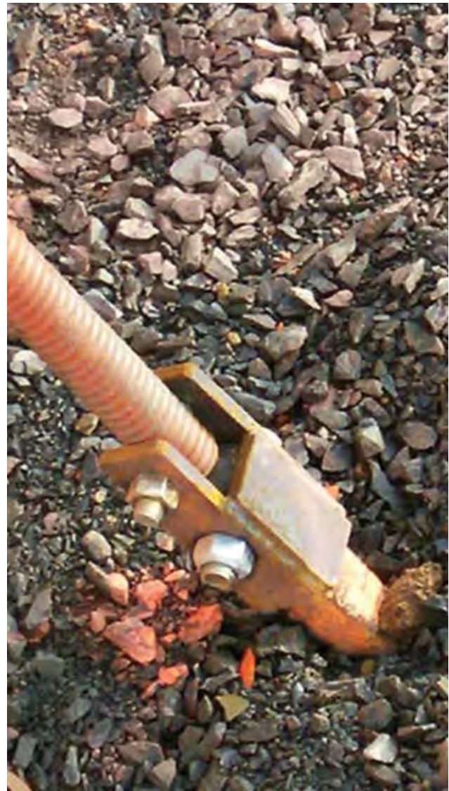
INCORRECT Brace-to-HGA Connection
