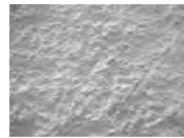
Fractured Concrete P/C 270583 0.090 mil Styrene P/C 270508 0.110 mil ABS
