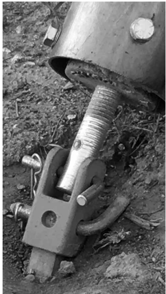
INCORRECT Brace-to-HGA Connection
