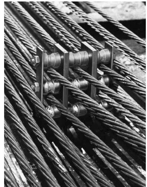
Illustration of swivel action as strand restraining device responds to strand tensioning.
