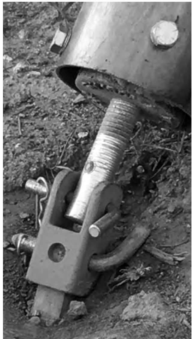
INCORRECT Brace-to-HGA Connection
