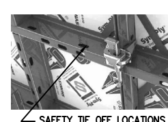
SAFETY TIE OFF LOCATIONS (DO NOT ATTACH TO CRANE)
