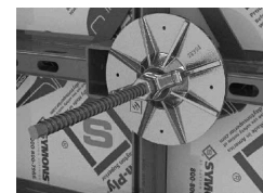
TYPICAL TIE PLATE ORIENTATION AT PANEL JOINTS
