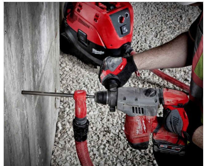
Hollow Vacuum Drill Hole Preparation
