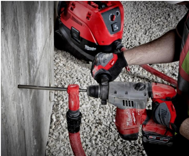
Hollow Vacuum Drill Hole Preparation
