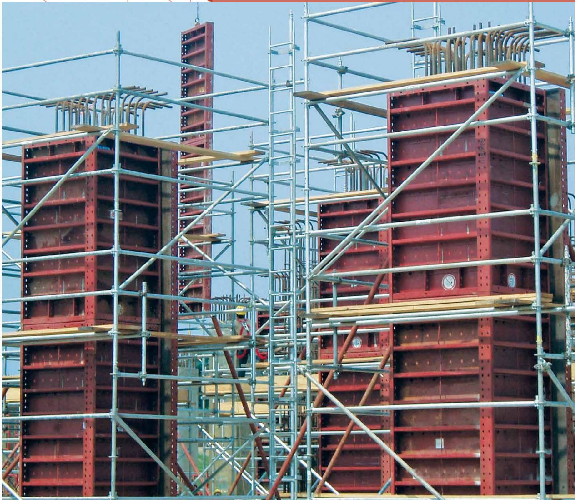
**PROJECT SHOWN:** Bechtel Oil, Gas and Chemicals utilizes Symons Adjustable Column Forms System on the first liquefied natural gas (LNG) storage and regasification plant in West Africa.
