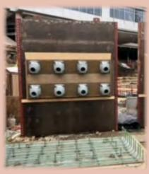
The Symons Engineering Group came up with a plan using Max-A-Form® STS forming system - along with 8" Versiform walers - to eliminate the need for those ties running the length of the beams.
