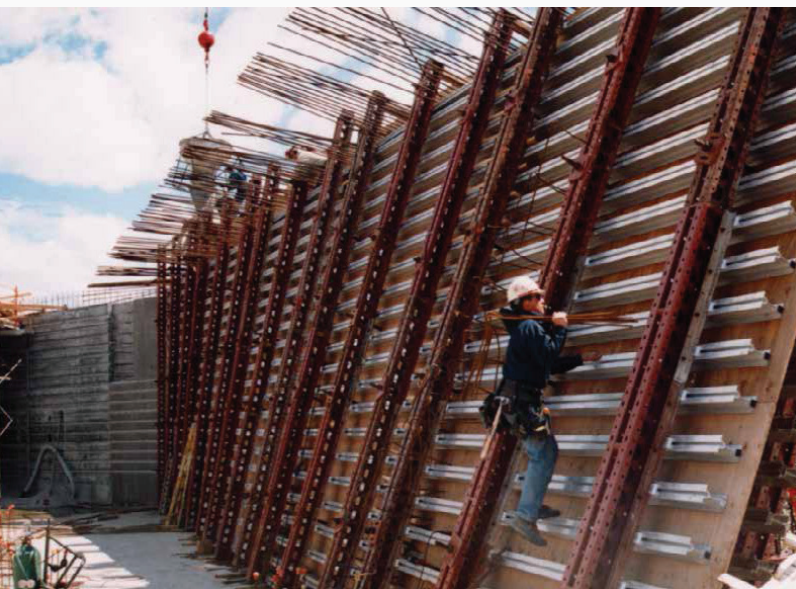
Symons Soldier was used as walers to carry the Taper Tie loads for the Aluminum Beam Gangs.
