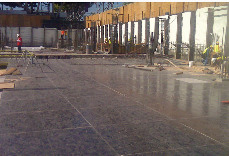
The system was erected at a rate of 160 square feet per manhour despite the crew not being familiar with it initially.
