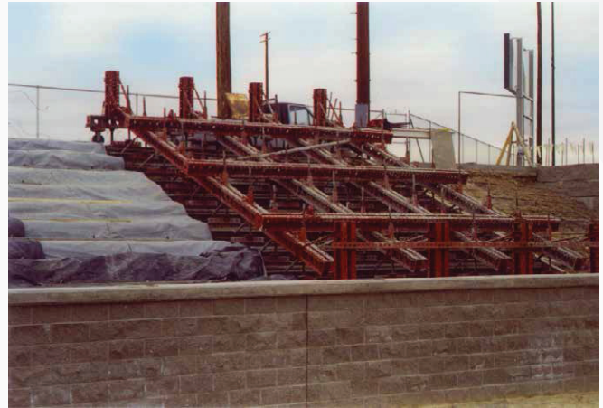
A grid of Symons Soldiers and Max-A-Form components supported the Steel-Ply forms for the high school stadium project.
