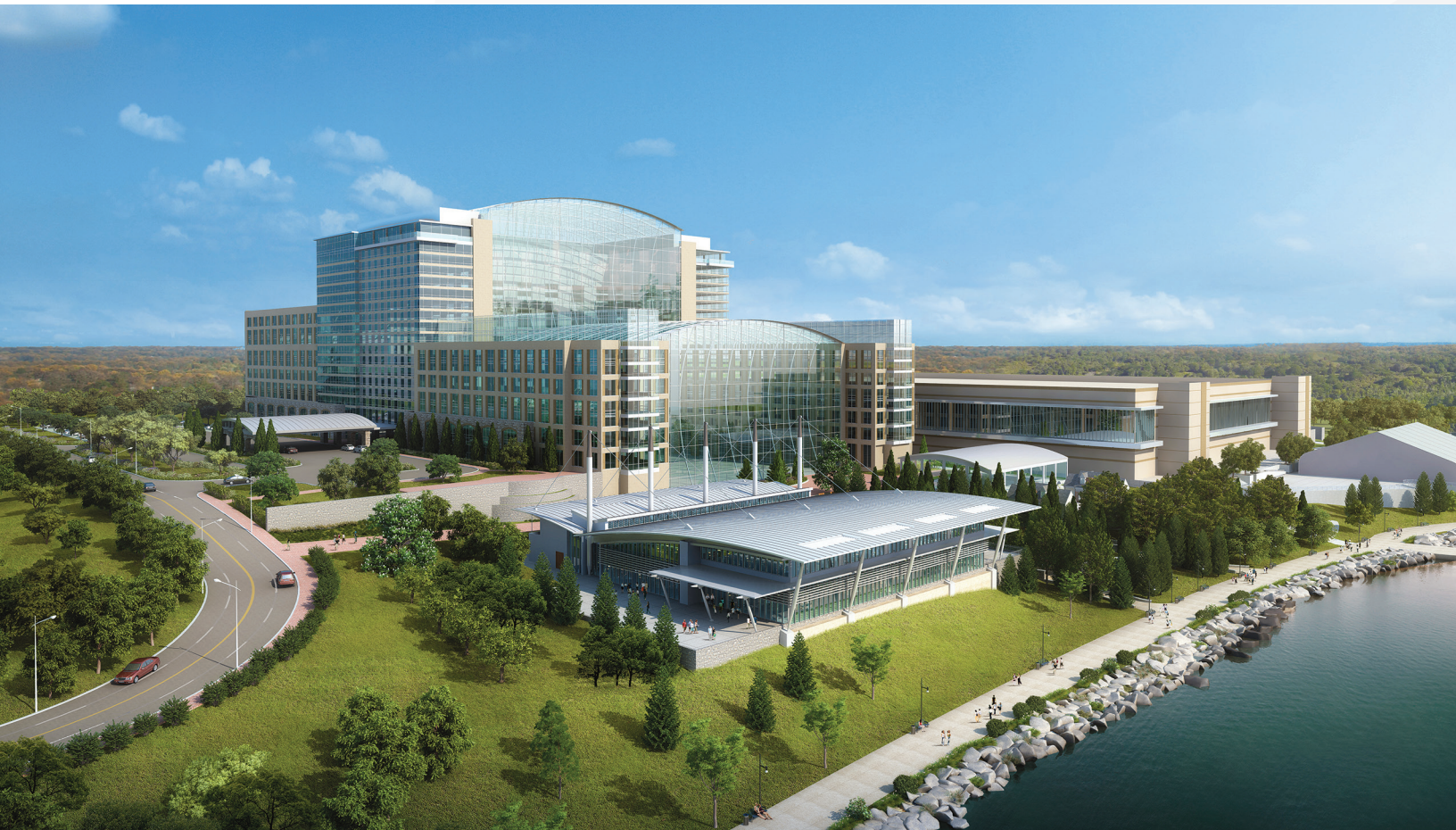
The luxurious Gaylord National Resort and Convention Center (above) is the centerpiece of the National Harbor project (right), just outside of Washington, D.C. (Rendering courtesy of Gaylord Hotels.)
