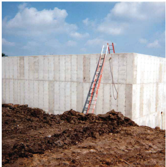
Steel-Ply forms were used in a handset application where muddy conditions did not allow them to place a large crane.
