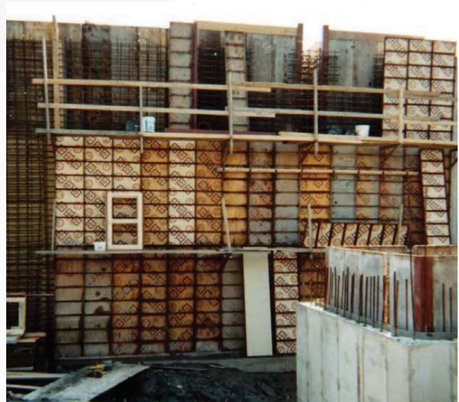
The Steel-Ply forming system was used for foundations and walls throughout this large expansion project.
