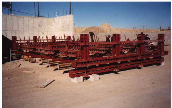
The 20' wide system was designed to roll from one location to another for multiple reuses.
