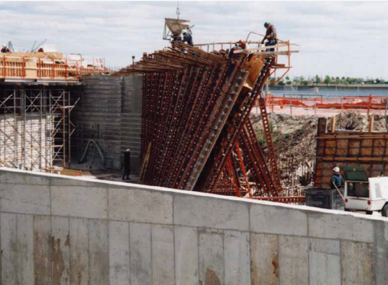
The concrete retaining wall was designed with a 25° twist that posed some unusual forming and support challenges.
