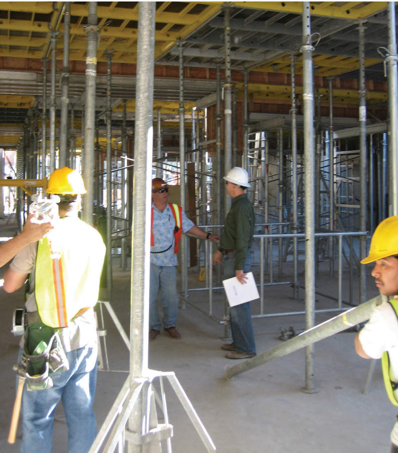
The small crew worked quickly, even at a forming height of twelve feet.
