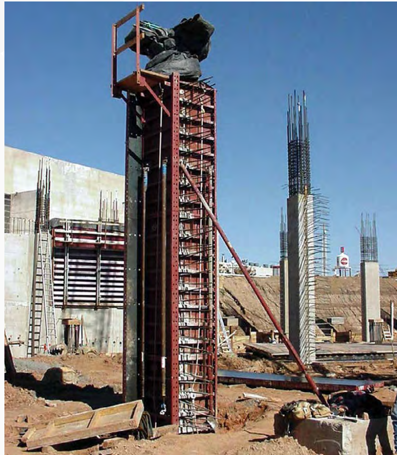
Adjustable Column Forms allow contractors to reconfigure the units and produce a variety of column dimensions with the same equipment.
