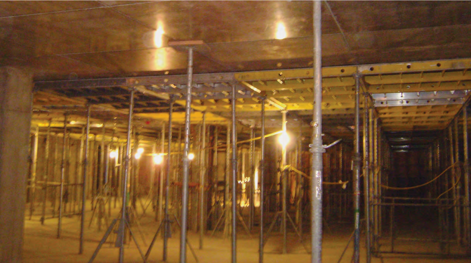
The composite-faced DeckFast panels produced an exceptional concrete finish.
