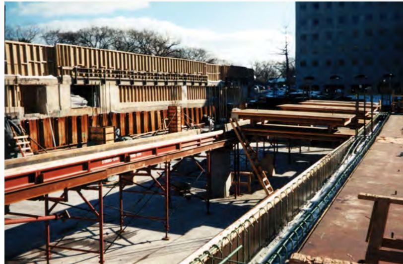
The pre-built deck panels span between the beam forms.
