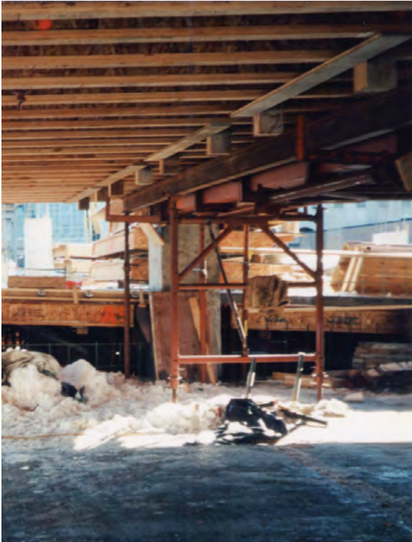
The strong and adjustable load frames with wide deck panels allowed large, clear work spaces for easy accessibility.
