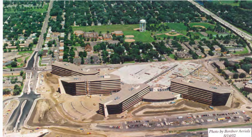
The two million sqft parking structure, one of the largest privately owned ones in the world, was the first time Opus used the Garage Beam System.
