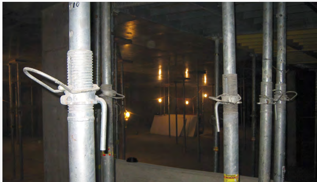
The design of the stripping pin allows a simple hammer blow to relieve concrete pressure from the shore, making removal fast.
