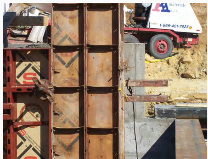
Standard Taper Ties can be used even when Steel-Ply is included in a project, simplifying inventory.
