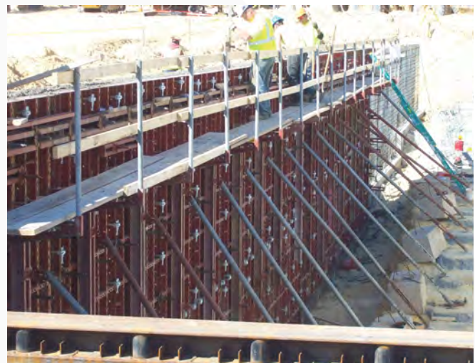
The Sym-Ply system includes a complete line of accessories, such as walkway brackets and braces.
