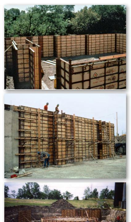
The Steel-Ply forming system is a pre-engineered, factory-built, reusable concrete forming system. It may be used in handset or gang form applications, for commercial or residential structures. The Steel-Ply forming system can form walls of almost any shape or size, with accessories for special structures and details. This system is more productive and economical than job-built plywood formwork or other forming methods.
