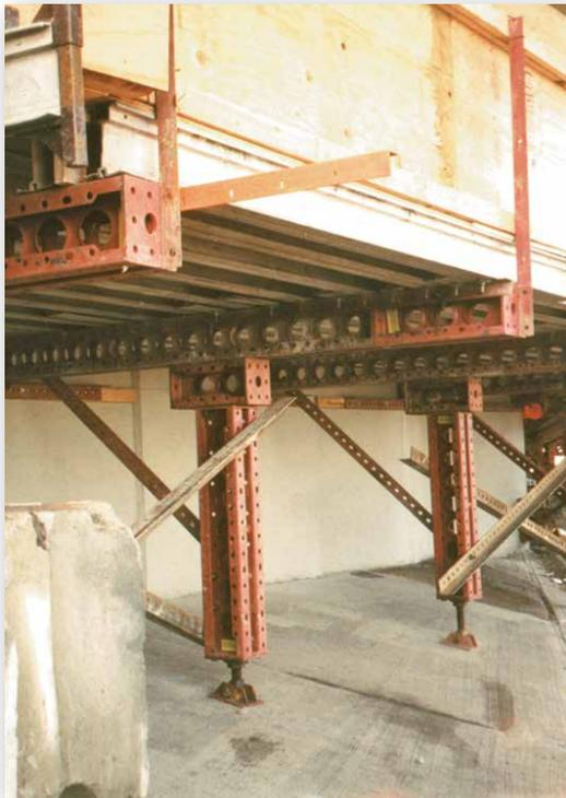
The Symons Soldier system is a lightweight, yet extremely strong, construction beam system with virtually unlimited application possibilities.
