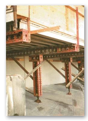
Symons Soldier beams permit bolting on all four flanges in addition to end and web bolt holes. The flange holes are a combination of holes and slots at 3" centers to provide dimensional adjustment and versatility.
