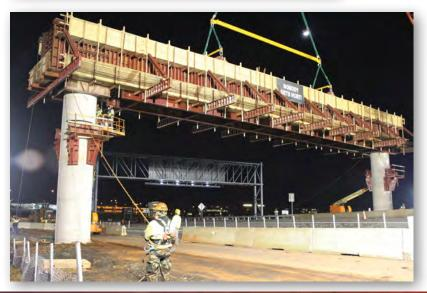
The Max-A-Form STS forming system is the Industry leader in rentable, self-spanning, steel formwork. Its superior pour pressure and moment capacities result in labor and material savings for the end user. The all-steel, welded frame make it the ideal choice for gang forming tall structural walls, pouring tieless columns, or for supporting concrete over long spans without shoring or custom equipment. The proprietary design and manufacturing process result in a superior finish, pour after pour.
