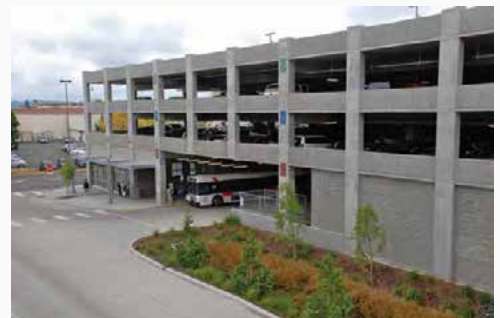
Clackamas Town Center Parking Garage Portland, Oregon
