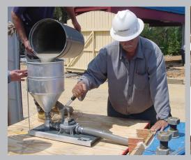
1107 ADVANTAGE GROUT is a non-shrink, non-corrosive, non-metallic cementitious grout. 1107 Advantage Grout is designed to provide a controlled, positive expansion to ensure an excellent bearing area. 1107 Advantage Grout can be mixed from a fluid to a stiff plastic consistency.
