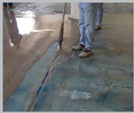
LEVELAYER® is a cement based, nonshrink, self-leveling floor underlayment designed for interior use. The LeveLayer provides a smooth subfloor that typically will accept floor coverings in as little as 14 hours after installation. Just mix with water, pour or pump, and it will seek its own level to produce a smooth, flat, hard surface.
