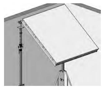
Hang the panel as shown. Make sure that the panel is hooked by the cams of both bearing devices. Hanging the panel requires two workers.
