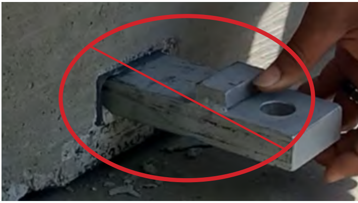
FIGURE 6 - Stopper bar NOT flush with PBA 10K void
