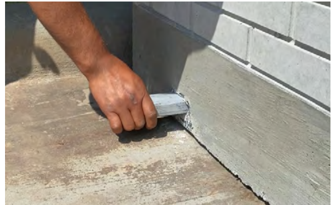
FIGURE 4 - Insert bar until stopper is flush with void
