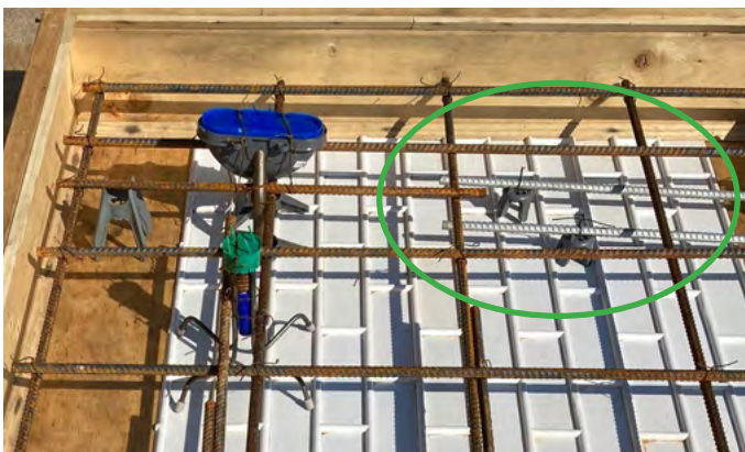
FIGURE 2 - Correctly supported with chairs
