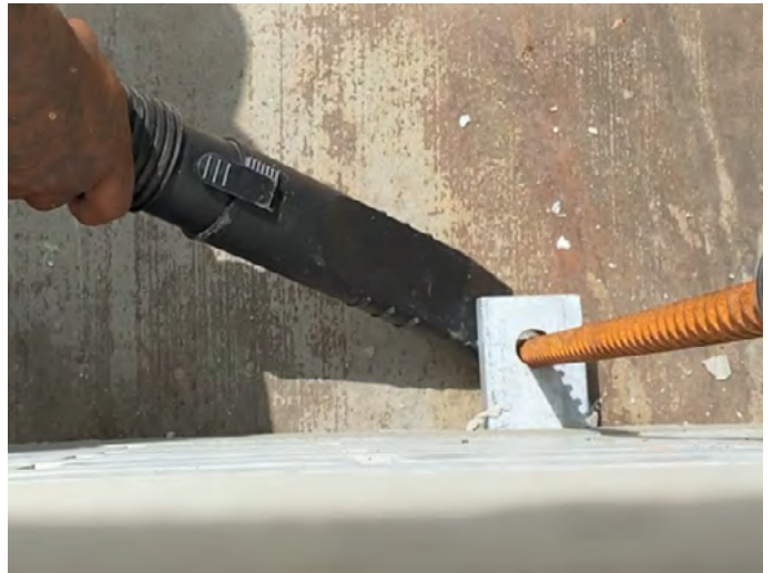
FIGURE 6 - Stopper bar NOT flush with PBA 10K void
