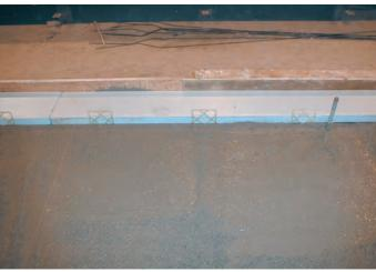
Delta Ties inserted into the first wythe - the exterior wythe along the edge of the second wythe — the rigid insulation.
