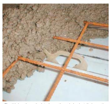
The third wythe — the interior wythe — being installed over the insulation, incorporating the Delta Tie and rebar.
