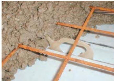
**Alternative Method:** Cut the first strip of insulation, then insert the first row of Delta Ties spaced vertically as required. Add the remaining courses of insulation and connectors. Foam-back tape is available for sealing the insulation joints, if necessary.
