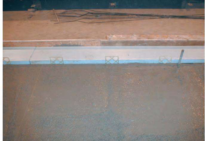
Delta Ties inserted into the first wythe — the exterior wythe — along the edge of the second wythe — the rigid insulation.
