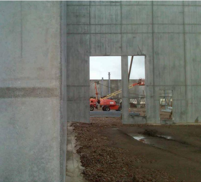
*The panels for this FedEx facility under construction in Philadelphia were braced by Accubrace Helical Ground Anchors (HGA) which helped them withstand the high winds and drenching rain from Hurricane Sandy.*
