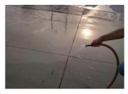
Be sure to keep the surface continuously wet with the Sure Hard Densifier J17. Do not allow the product to dry, apply additional product if needed to keep wet while working.
