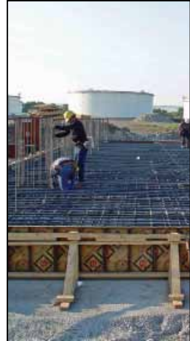
A new rail facility, electrical substation and control room featured concrete.
