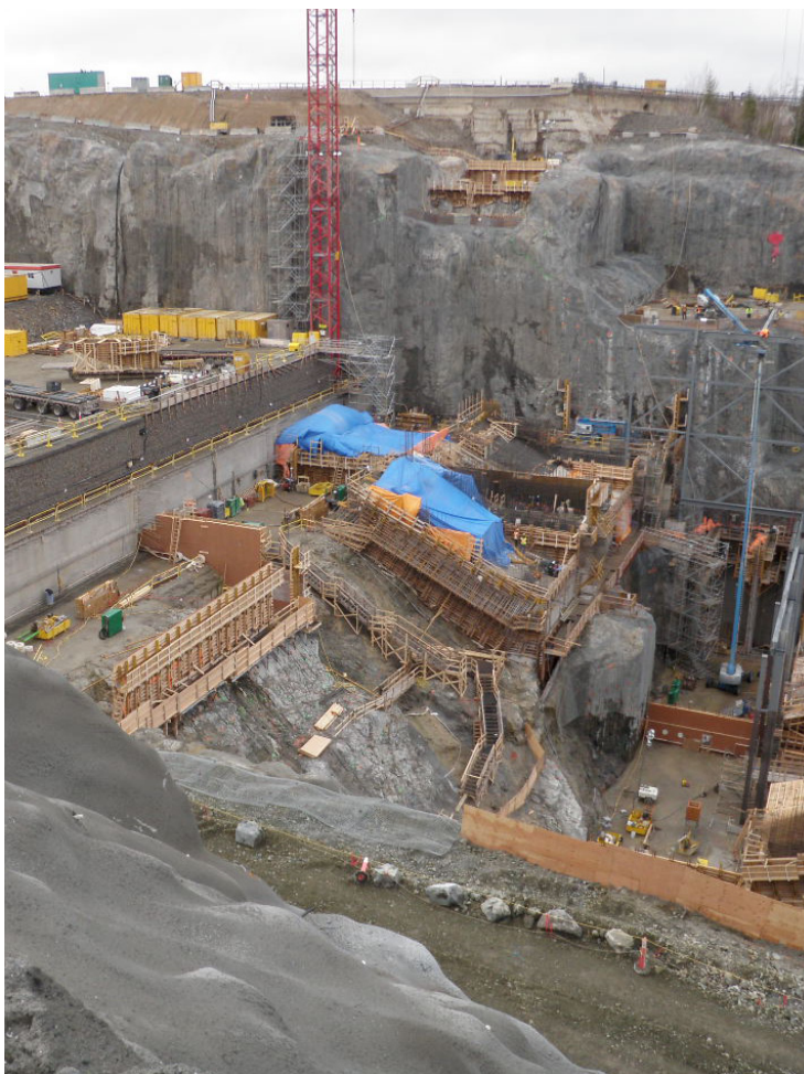
Construction of the Smoky Falls Intake occurring in November 2011
