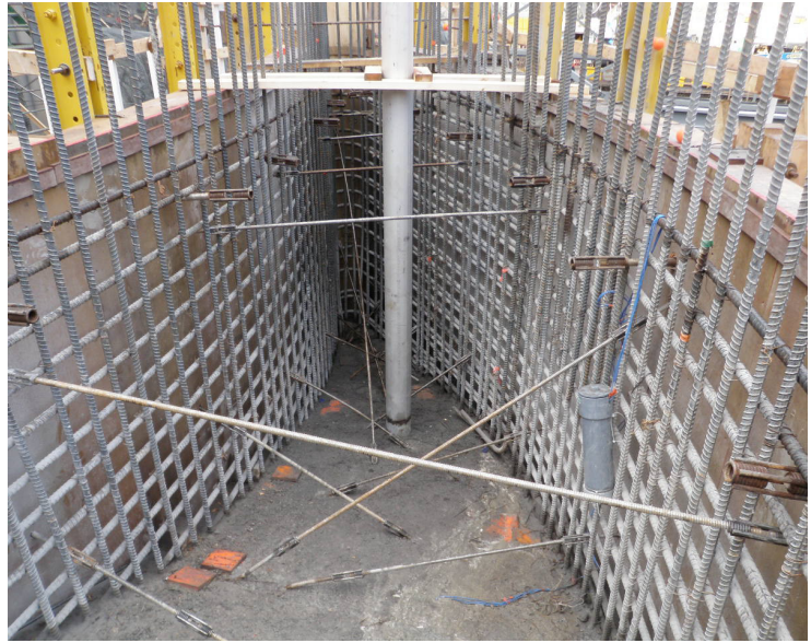
The intake pier nose utilized Dayton Superior products.
