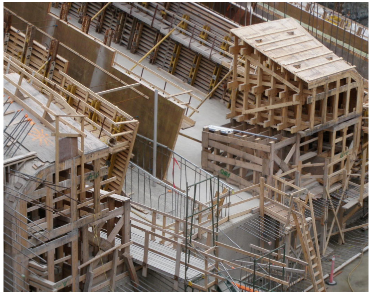
A closer view of the Smokey Falls Intake jobsite.
